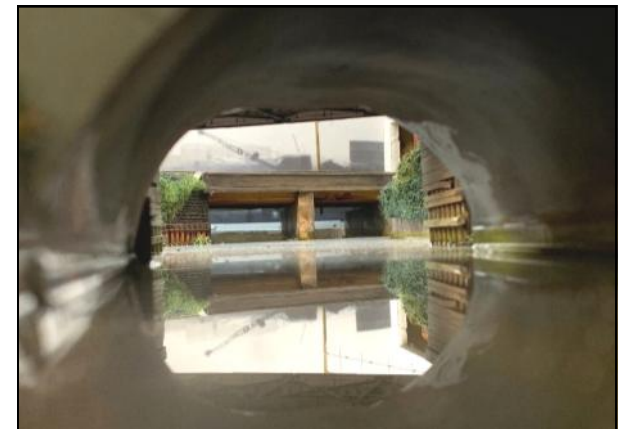
The view under the bridges, Pennsylvania RR Bridge and the Joseph Berliner Co. Bridge.
