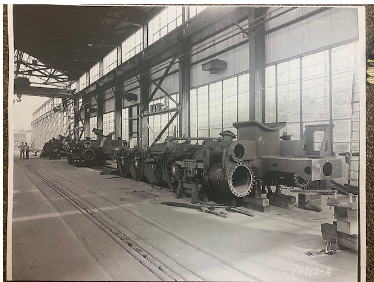
Interior of Vulcan Assembly Building
